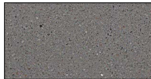
BROOM FINISH CONCRETE FLOOR
